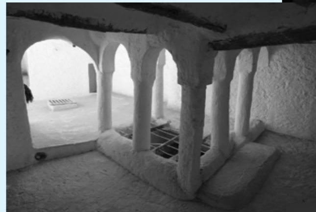
Inside Mozabite House, Residence of André Ravereau. Arcades Supporting the Terrace
