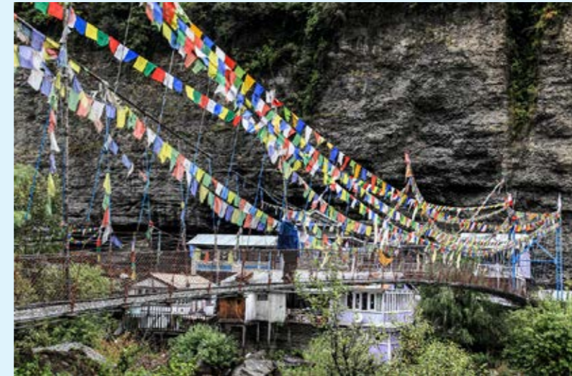
Hanging bridge, Pisang
