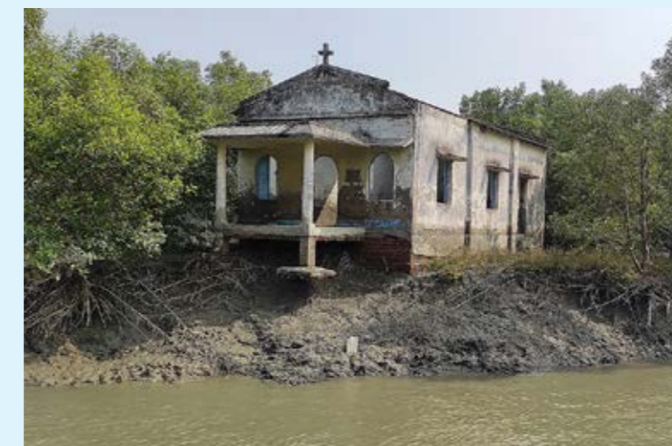
Church After erosion
