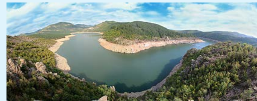
Arda Kardzhali Dam Rope Bridge
