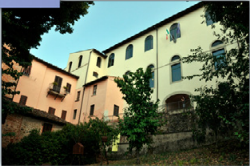
The beautiful and impressive building hosting the FIAP Exhibition Centre in Montevarchi
