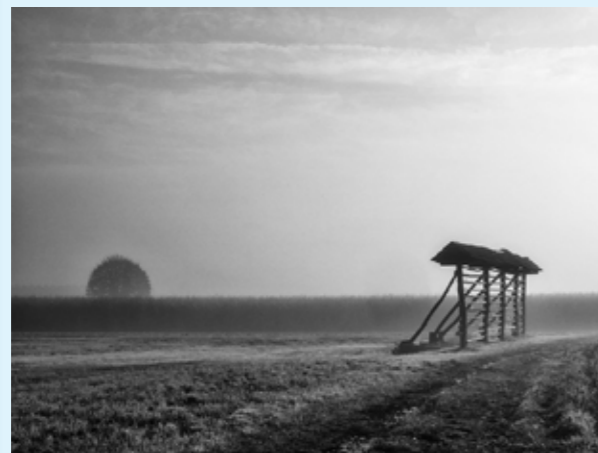
Initially the hayracks were completely made from wood pillars, bars and roofs. In more recent years the pillars have been made of concrete and for the rooves they used several man-made materials
